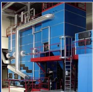
The Danstoker horizontal and vertical bio-fuel boilers are fire-tube boilers, and if required combined with water-tube sections. Capacities ranging from 200 kW to 24,000 kW or 40 t/h steam up to 86 barg.
